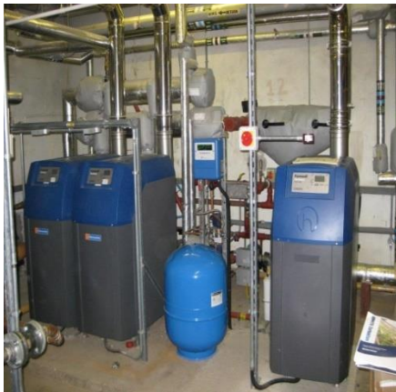
Installation of efficient condensing boilers
